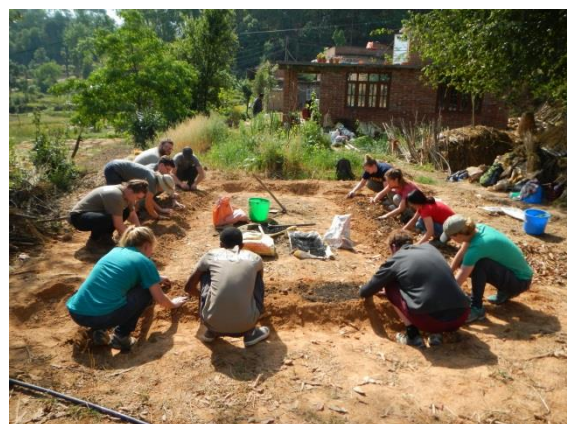
Amending the topsoil of all the protective berms (Nepal, April 2016)
